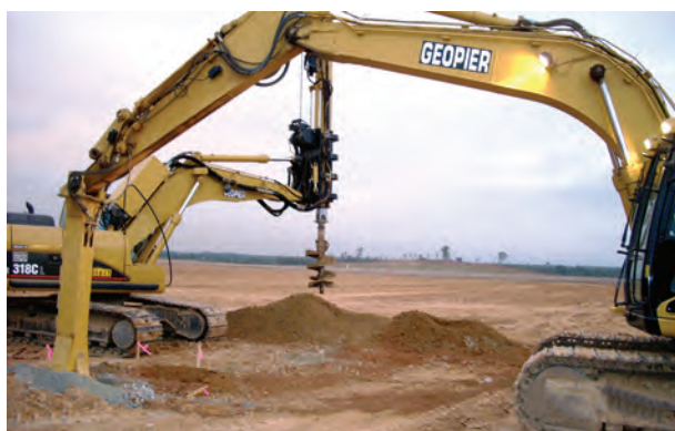
KIA Manufacturing Plant Construction West Point, Georgia, USA
