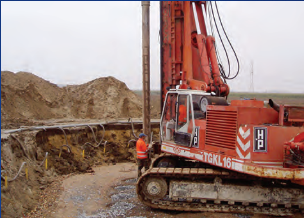
Wind Park Construction Purzien, Germany
