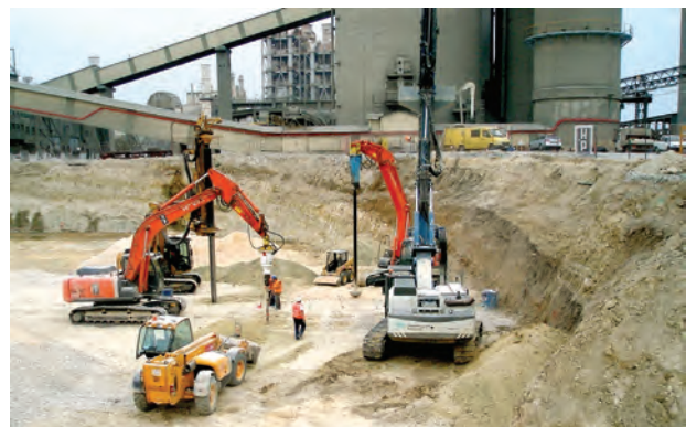
Cement Clinker Dome Construction Medgidia, Romania
