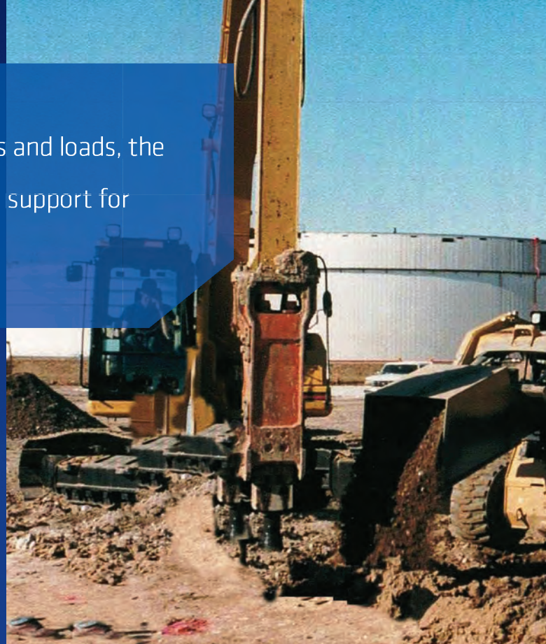
Houston Fuel Oil Terminal Company Tank Yard Construction Houston, Texas, USA
