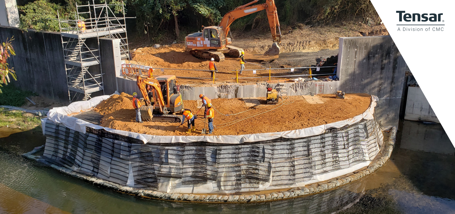
RSS being constructed within a limited working space.
